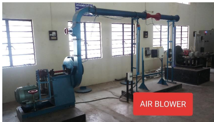
Fig. 2 Air Blower Equipment
